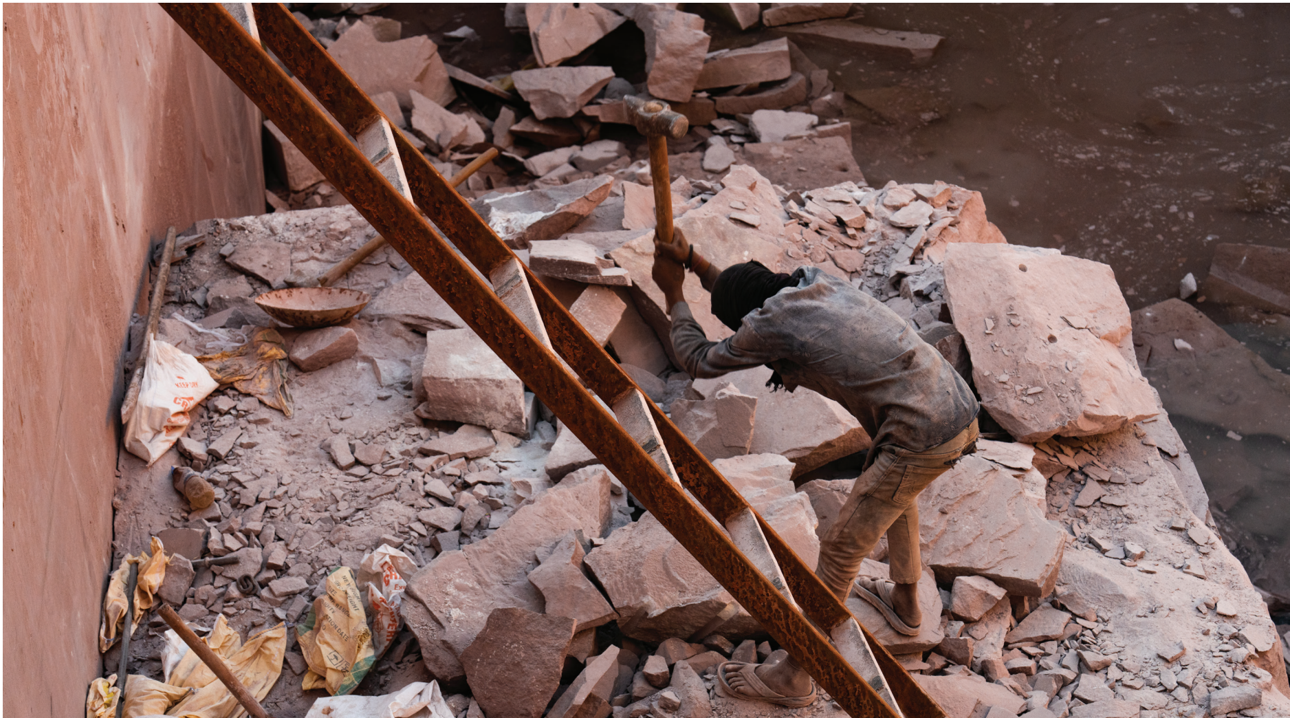
Workers breaking stone are exposed to dust that is linked to serious lung diseases. Photo © Siddhartha Joshi
