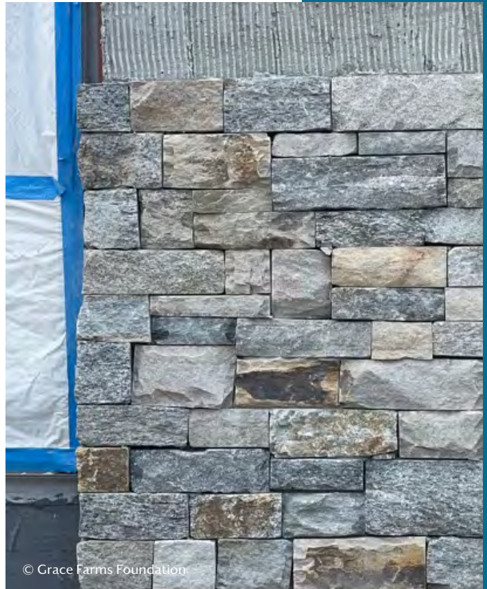
Installation of natural stone facade
